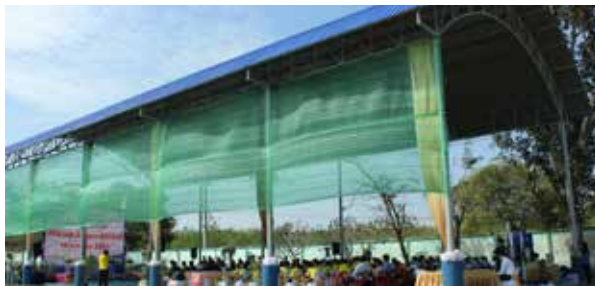
Steel Dome Project in Thailand
