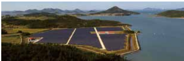
POSCO Energy's Sinan Solar Power Generation Complex (third phase)
