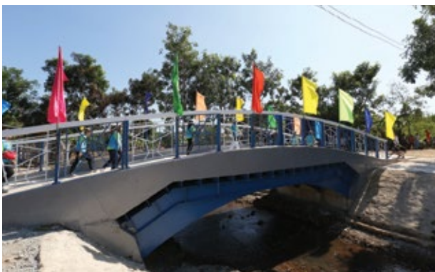
↑ Steel bridge built with POSCO steel
