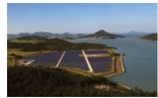
↑ POSCO Energy's Sinan Solar Power Generation Complex (third phase)
