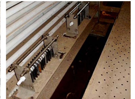
Installation of specimen rack in GGH preheater
