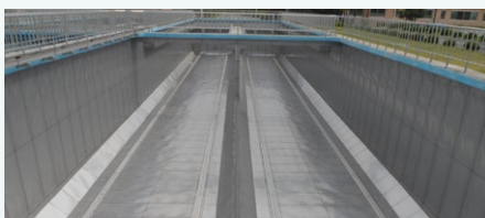
Applied STS329LD to the lining of the sedimentation tank at a water purification plant.
